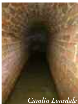
Camlin Lonsdale Old sewer under the House terrace
